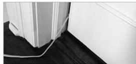
At loose electrical connections or cords damaged by doors closing on them
